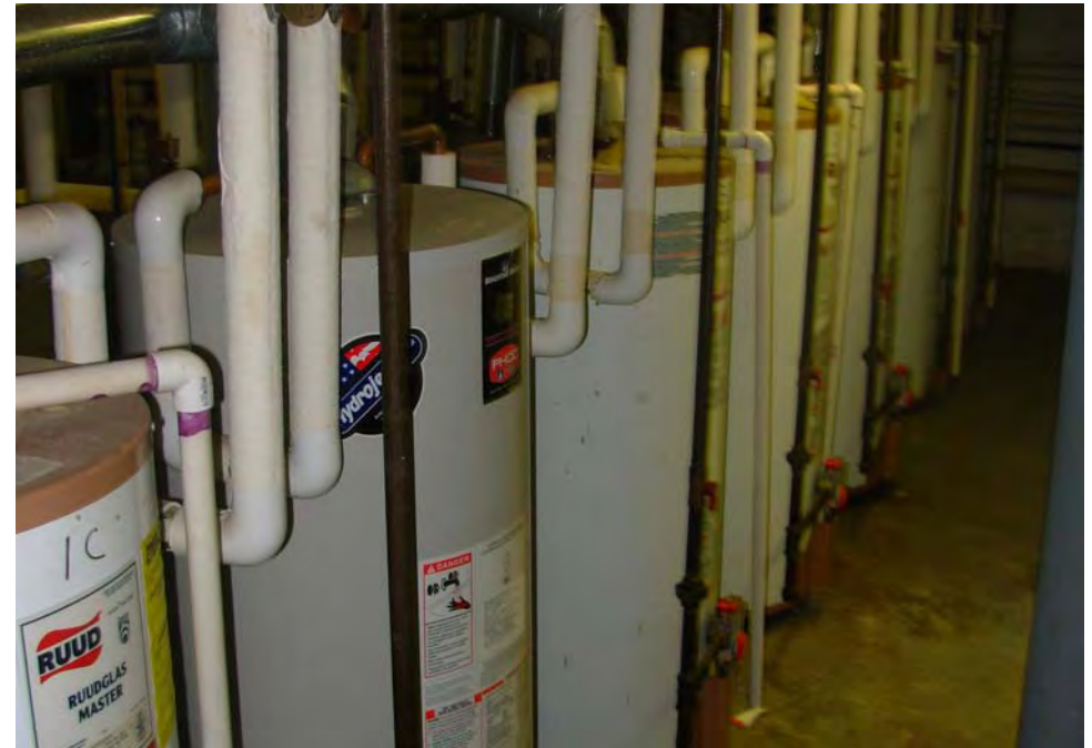
20. Typical unit DHW tanks
