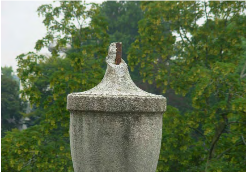
9. Architectural elements exhibiting deterioration, note protruding rebar
