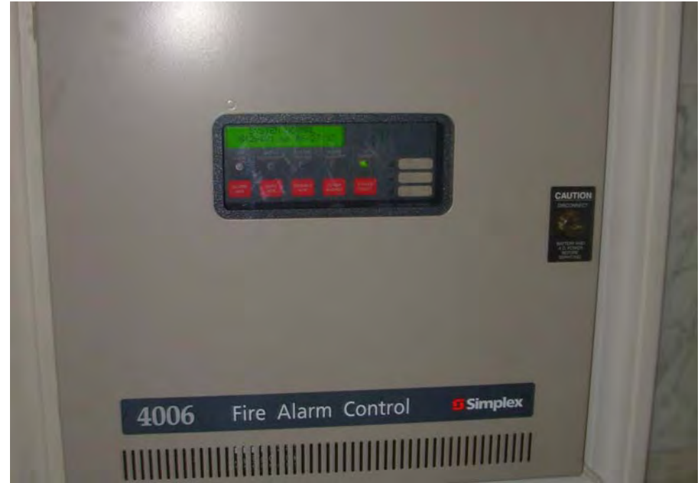
22. Typical fire detection monitoring panel
