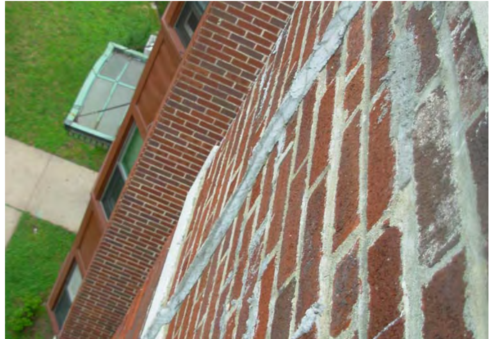
10. Recent masonry repairs at upper front elevations
