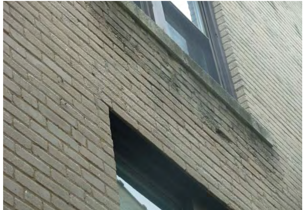
8. Spalling masonry and mortar deterioration
