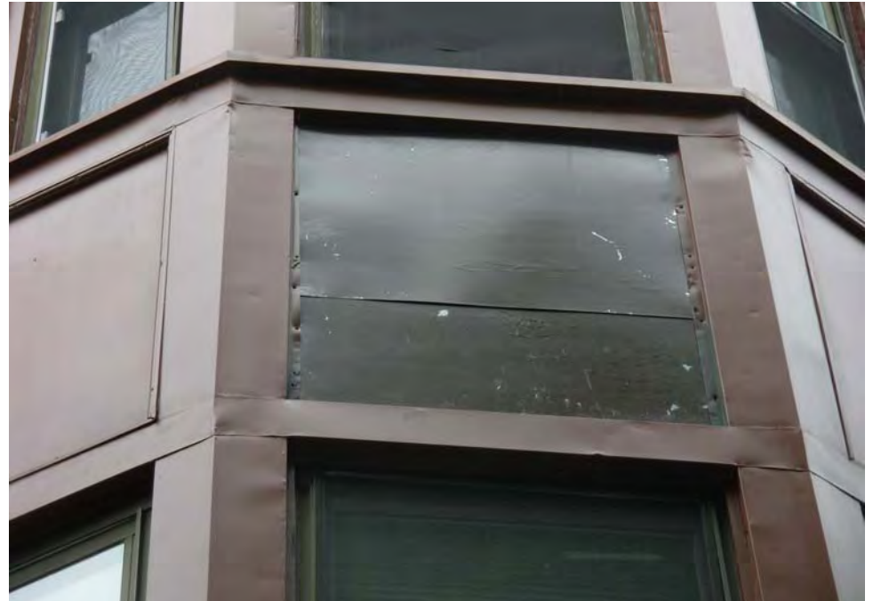
6. Metal infill panels at window bays
