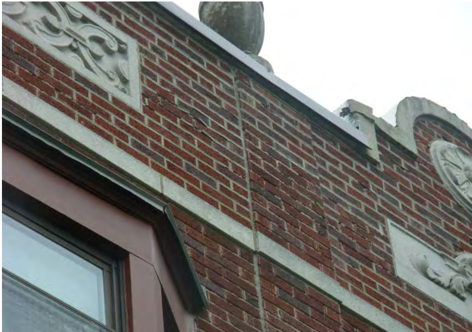
7. Mortar deterioration at sections of upper front walls
