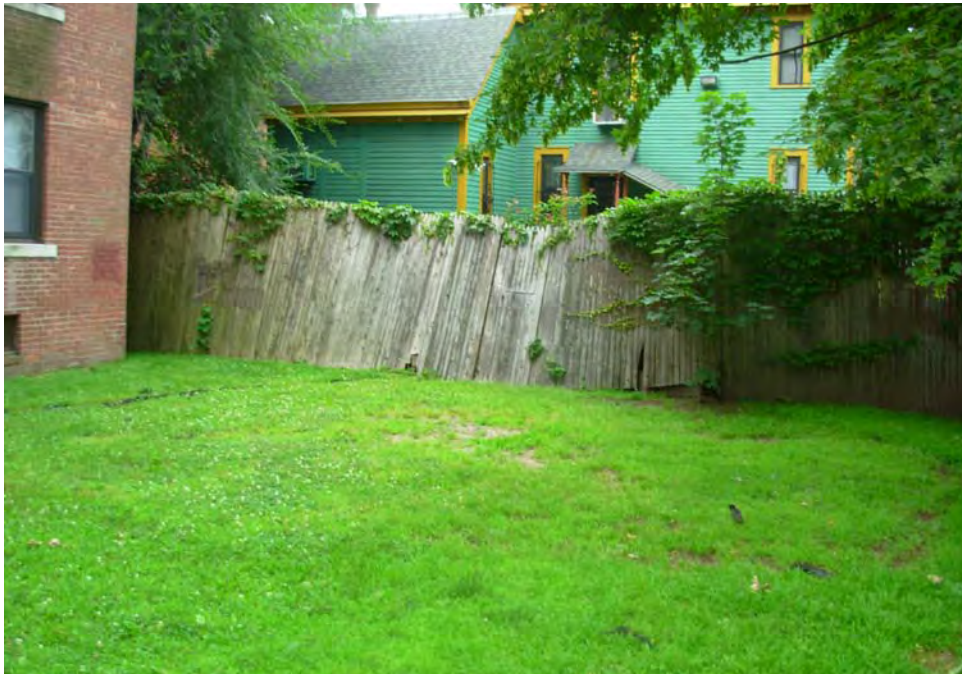
3. Wood stockade fencing damage and leaning conditions
